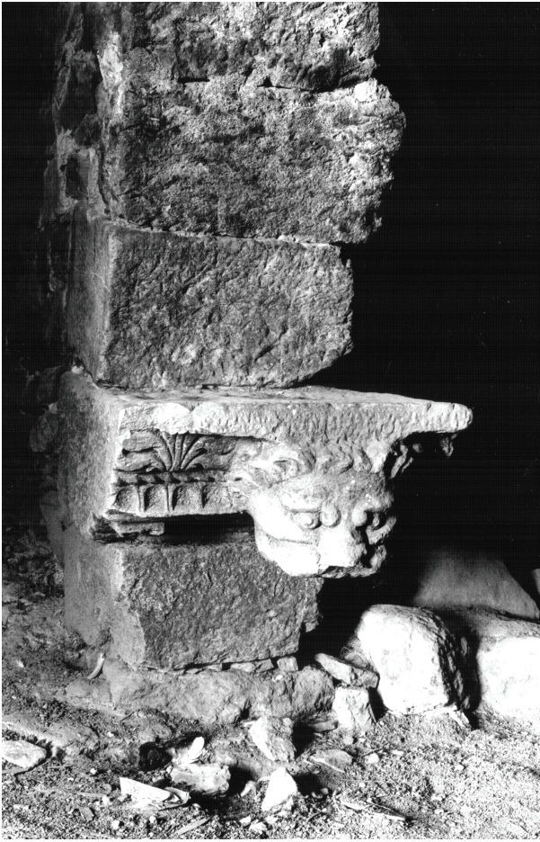
Figure 1.7 Al Qasr: arch springer reusing a lion carving from a Nabatean temple.
