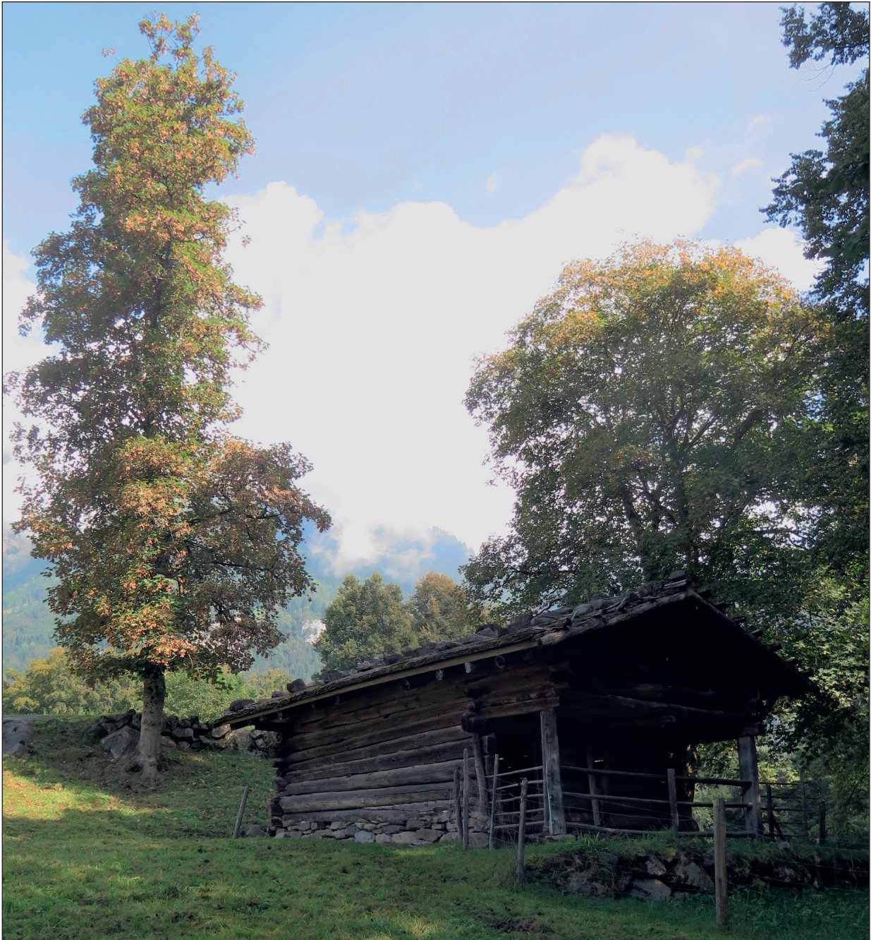
Figure 1.4: This summer hut, now rebuilt at the Ballenburg open-air museum at Brienz, Switzerland, was first erected in 1520 in the Litschen valley, Axalp at 1850 m. (6070 feet) a. s. l. It had no internal divisions, and the sleeping chamber was in the projection over the entrance, which created a sheltered space beneath, where a cow could be milked. The archaeological signature would be a simple rectangular stony bank. (Photograph: Pete Herring)
