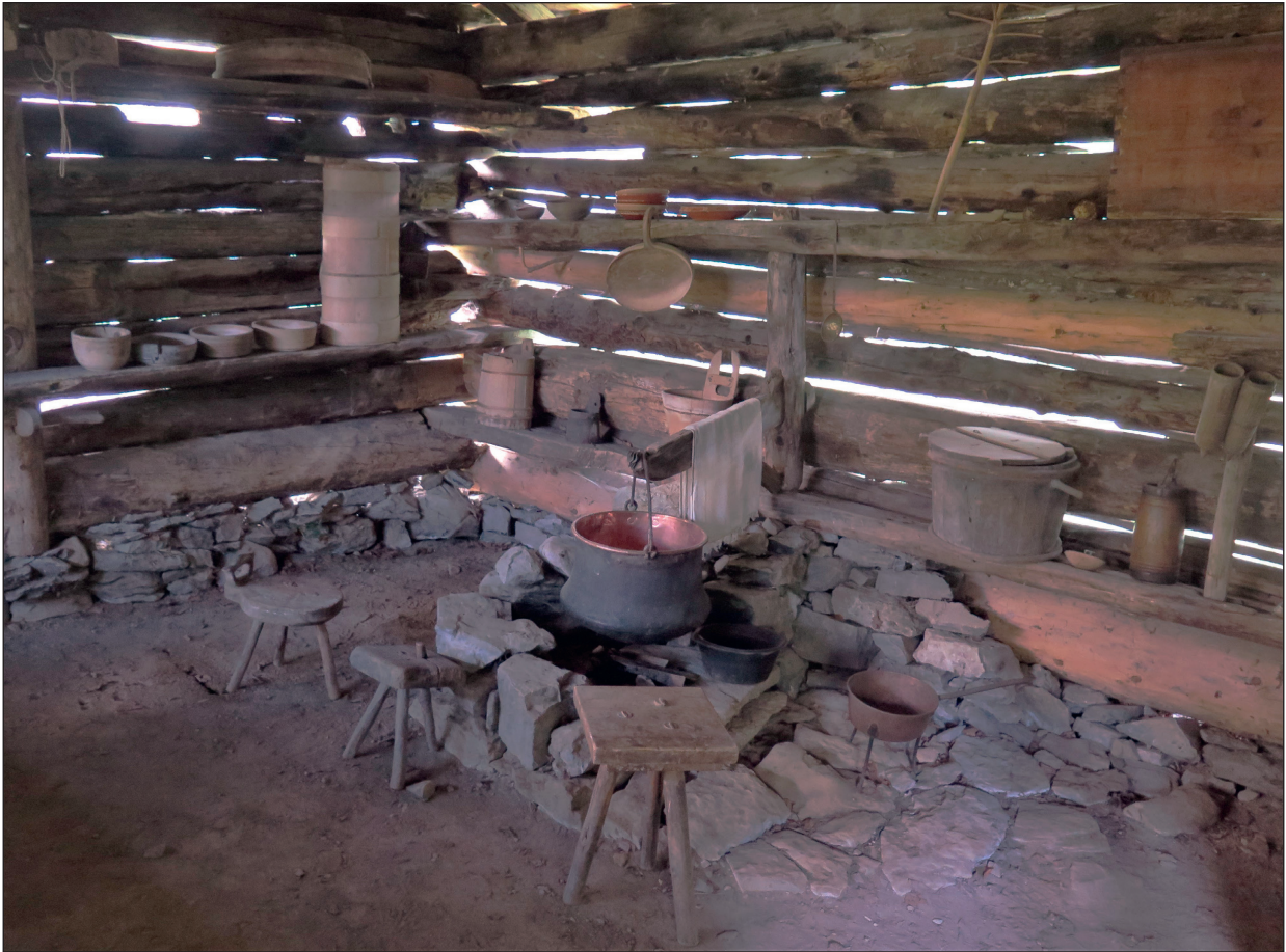
Figure 1.5: Interior of the Litschen Valley summer hut shown in Fig 1.4, showing the simplicity and flexibility of arrangements, which were focussed on the fire and the copper cheese-making kettle on an arm fixed to a rotating spindle that allowed it to be swung over and away from the heat. (Photograph: Pete Herring)
