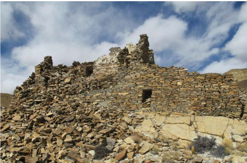
Figure 1b.5. One of the many hybrid structures built with both all-stone corbelled and wooden roofs in the stronghold of Dar sgam mkhar (c. 4250 m elevation), Gu ge.
