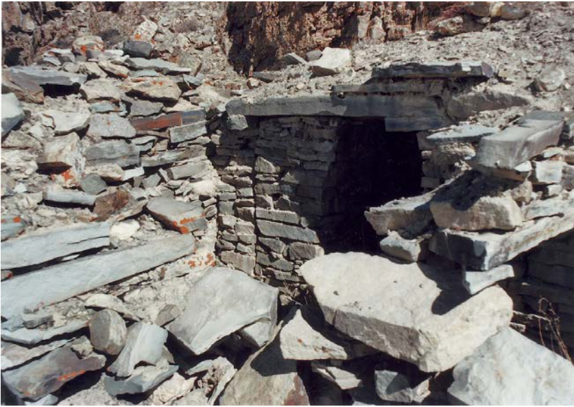
Figure 1b.6. The all-stone corbelled stonework of structures in the upper tier of the upper edifice, East complex, Sman bla pho brang South (5080 m elevation). The site is perched above a tributary valley of the Mount Kailash pilgrim's circuit, Spu rang.
