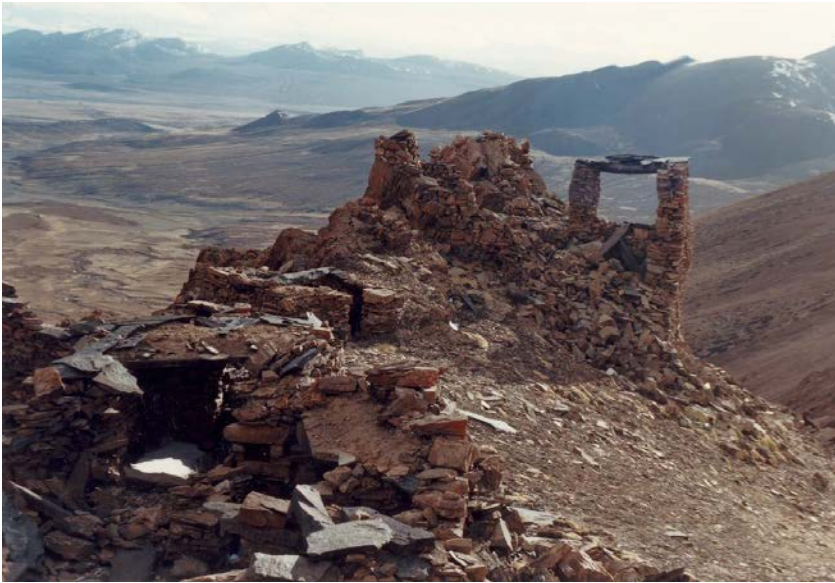
Figure 1b.4. All-stone corbelled residential structures in the west portion of the middle complex of a citadel called Jo mo ri rang mkhar (5060 m elevation), Spu rang.
