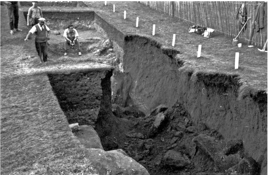
2.10. A lesson for all archaeologists who do not shore up the sides of deep trenches: the Thetford Castle trench collapsed just after we had climbed out for a coffee break (M37).
