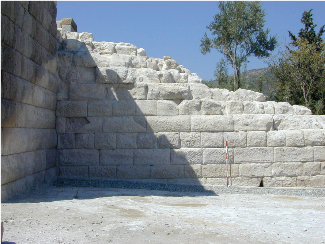
Figure 8: North wall of the gate-yard of the Myndos Gate at Halikarnassos (photo: P. Pedersen).
