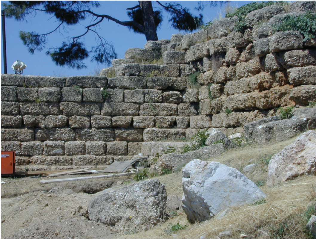
Figure 6: Retaining wall west of the Odeon of Pericles at Athens (photo: P. Pedersen).
