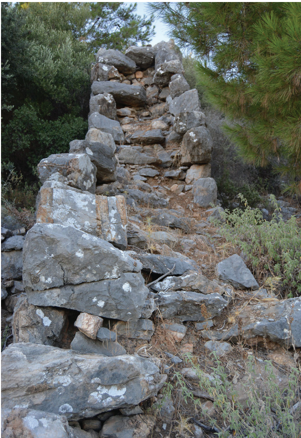
Figure 9: Rough drystone wall. City wall at Halikarnassos (photo: P. Pedersen).
