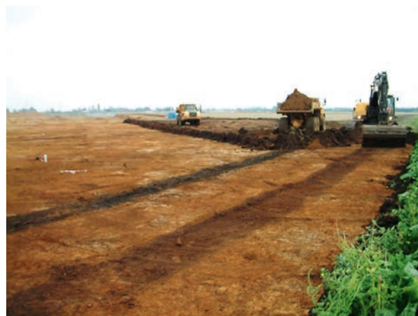
Plate 2 Machine removal of topsoils across the Site.
