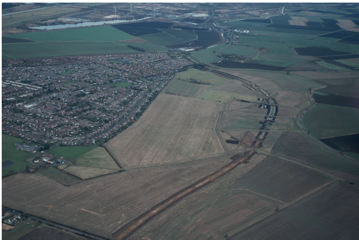
Figure 1.9. Bypass East stripped, looking north-east
