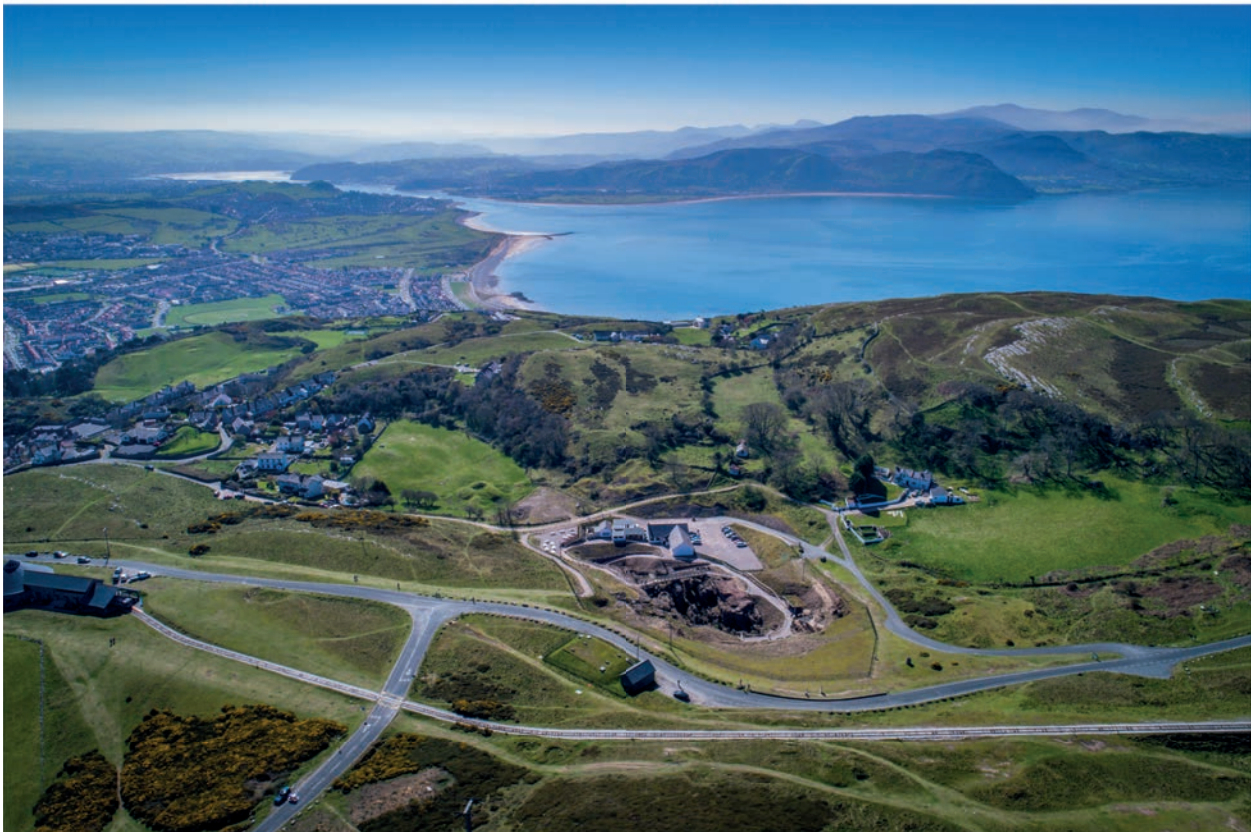
Figure 1.1: General aerial views of the Great Orme mine looking SE (top) and SW (bottom)(Great Orme Mines)
