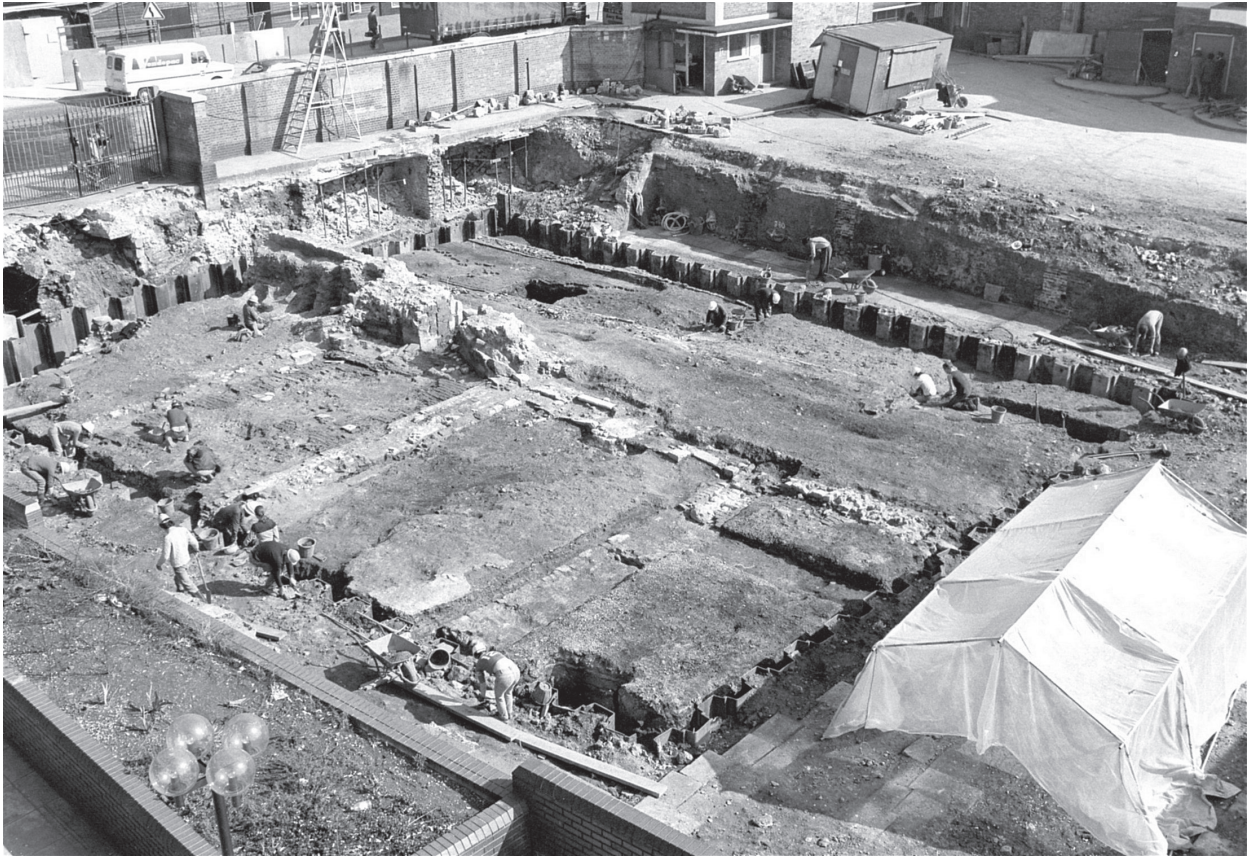
Figure 22 Site D (Billingsgate): the site after initial cleaning in 1982, showing the outline of pre-Fire buildings largely covered with debris of the Great Fire. These deposits were directly beneath the 19th-century buildings, the cellar walls of which, surrounding the excavation, were used to retain the upper 3m of strata. The cofferdam was designed for the archaeological project
