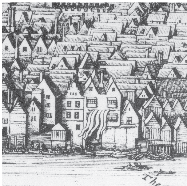
Figure 7 Detail from the panorama of 1647 by Wenceslaus Hollar, showing cloths hanging from poles on a building on the waterfront side of the Swan Lane (site A) site, probably part of a documented rebuilding of the property in or after 1638 as a house and dyeing establishment. The archaeological excavation took place in the area of buildings behind the waterfront
