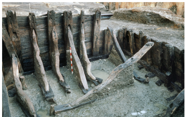
Figure 1 The early 13th-century waterfront excavated on the Billingsgate site, 1982, looking north from the river side. The section of revetment on the left (D:Waterfront 14), dated by dendrochronology to about 1235, was later conserved and displayed in the Medieval Gallery of the Museum of London
