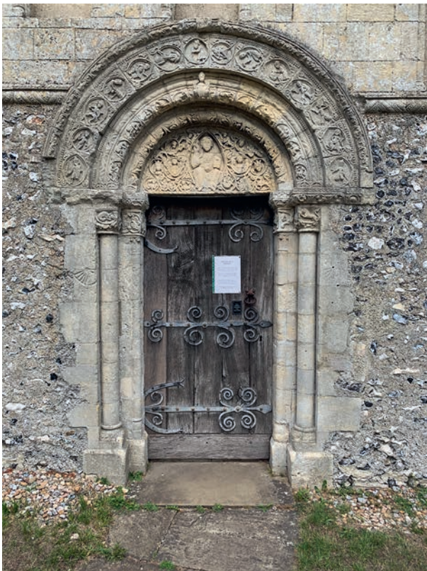
Figure I.3, Barfreestone, south doorway
