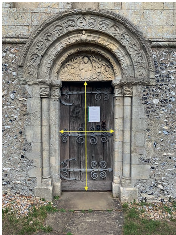
Figure I.6, Method for Doorway Measurements
