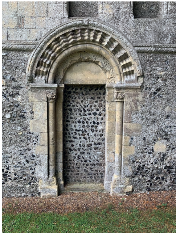
Figure I.4, Barfreestone, north doorway
