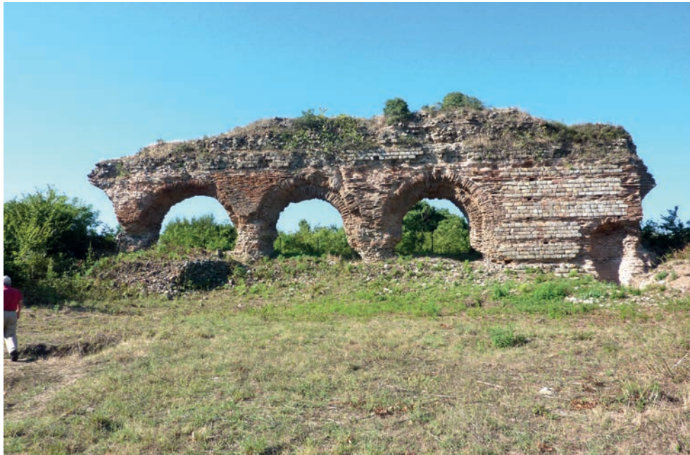
Figure 4. Aqueduct (photograph courtesy of Ş. Yıldırım).
