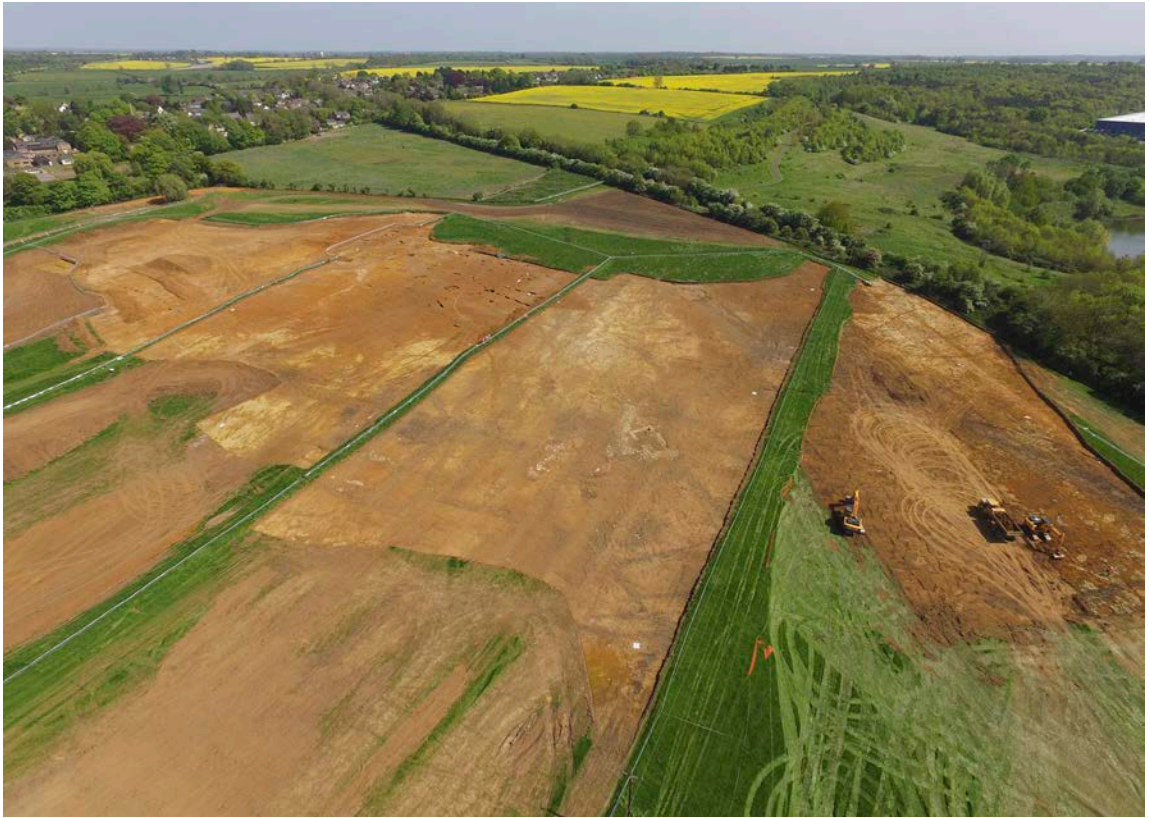
Figure 1.6 Initial machine strip of the excavation area nearing completion, looking south-east
