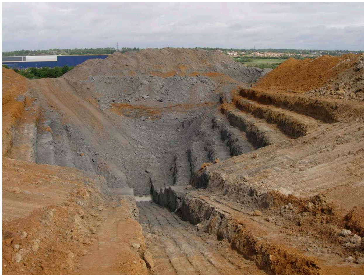
Figure 1.2 Engineering excavations in the Stage 1 area following completion of the archaeological works, shows the broad geological stratification, looking north
