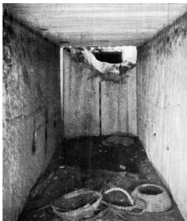
FIGURE 290 THE CLOSED PORTCULLIS IN THE WESTERN CORRIDOR OF THE BENT PYRAMID LOOKING WEST, WITH THE ROBBERS' HOLE IN ITS UPPER HALF. (FAKHRY 1959, PL. X.A)
