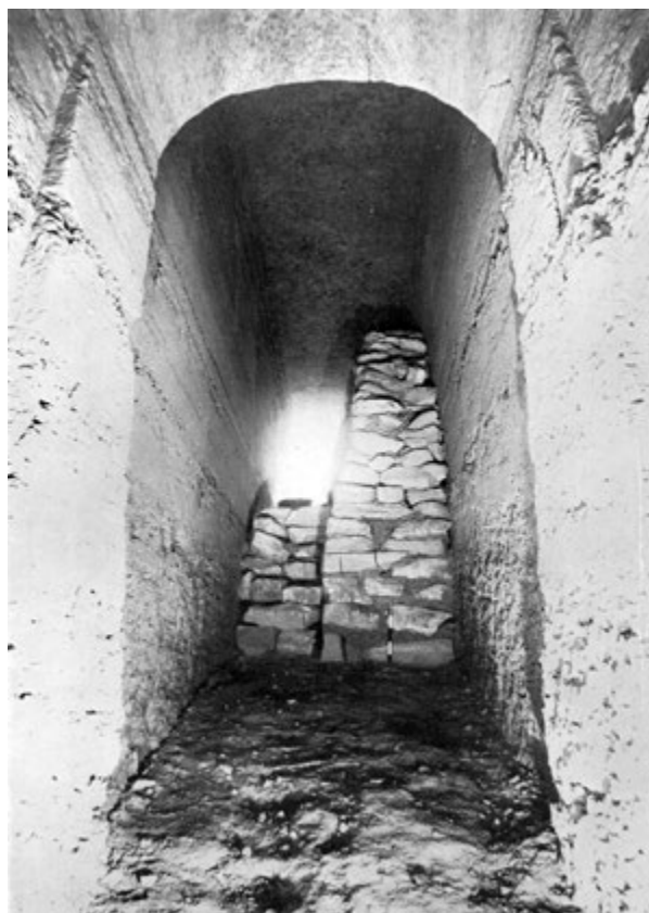
FIGURE 276 THE MASONRY ENTRANCE BLOCKING OF THE DESCENDING CORRIDOR OF THE PYRAMID OF SEKHEMKHET LOOKING NORTH. (GONEIM 1957, PL. XXI)
