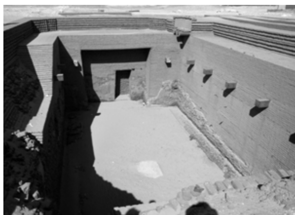
FIGURE 33 . THE RESTORED BURIAL CHAMBER OF THE TOMB OF KING DEN, SHOWING THE ENTRANCE AND THE BEAMS THAT SUPPORTED THE SHRINE AND ROOF. (PHOTOGRAPH BY THE AUTHOR)
