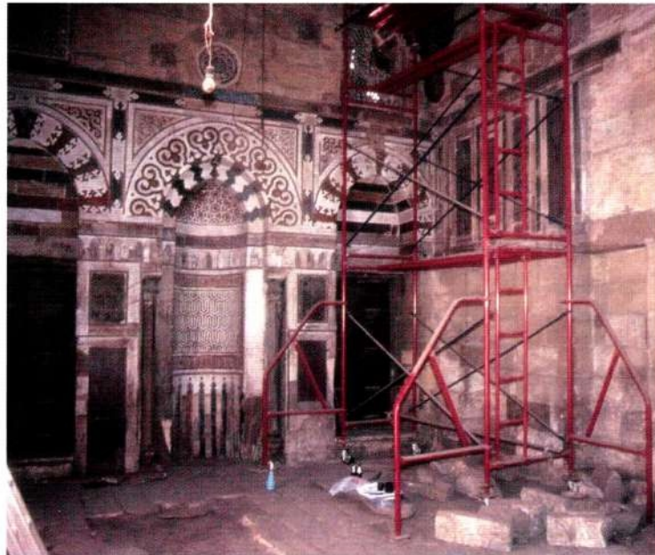
East (left) and south (right) walls of the Zawiya of Farag ibn Barquq. Photo: James A. Harrell
