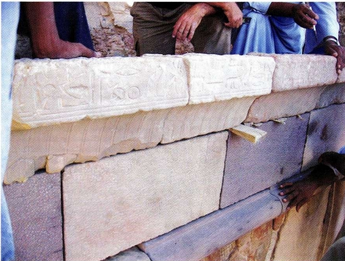
Cavetto cornice during installation. Photo: E. Pischikova
