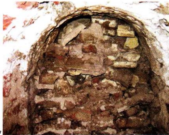
Figure 7. The left niche contained many fragments of limestone paving as well as bricks.
