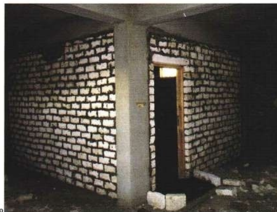
9. The beginnings of the "Mummy Room" during early construction phase.
