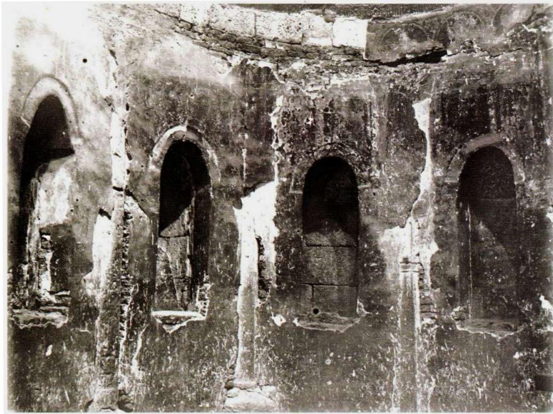
5. Eastern lobe of the Sanctuary, White Monastery Church, showing the Medieval brick and plaster walling up of the sculpted surface. Decorative motifs are visible in the upper right of the photograph. Photo: the Comité. Courtesy of the Musée du Louvre.
