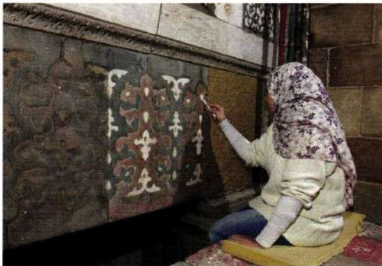
11. Marble decoration was cleaned both mechanically and chemically. A conservator is removing dirt from a surface first treated with chemicals applied in poultices (right). The darkened part to the left shows condition before conservation. Photo: Matjaž Kacicnik
