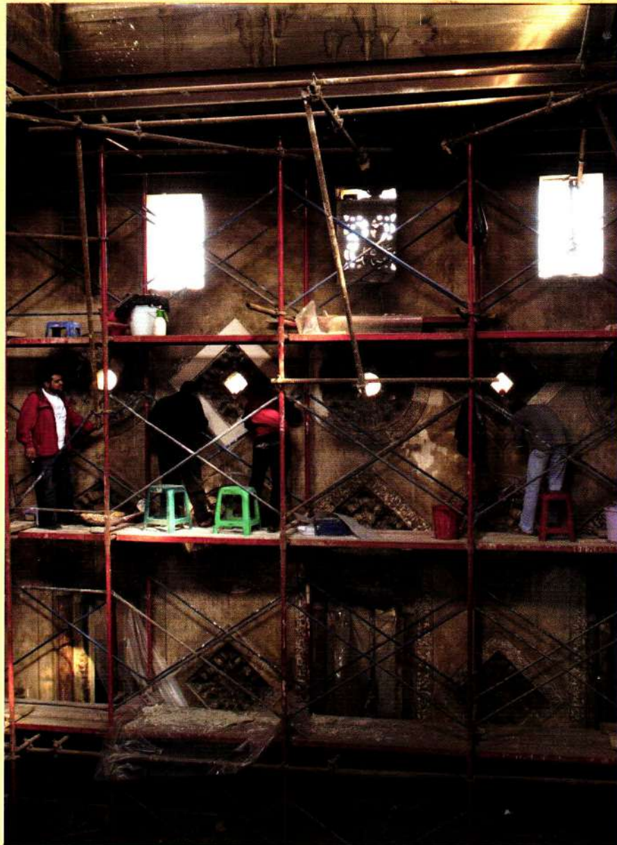
The manual cleaning of the intricate stucco decoration was a challenging and labor-intensive task. Photo: Matjaž Kacianik
