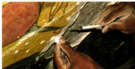
Re-attaching fragments in their original positions on the wall. Photo by Katherine Blakeney
