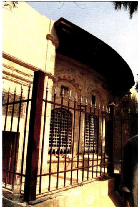
Sabil Hasan Agha Arzinkan before and after the completion of the conservation project. Photo by Nairy Hampikian
