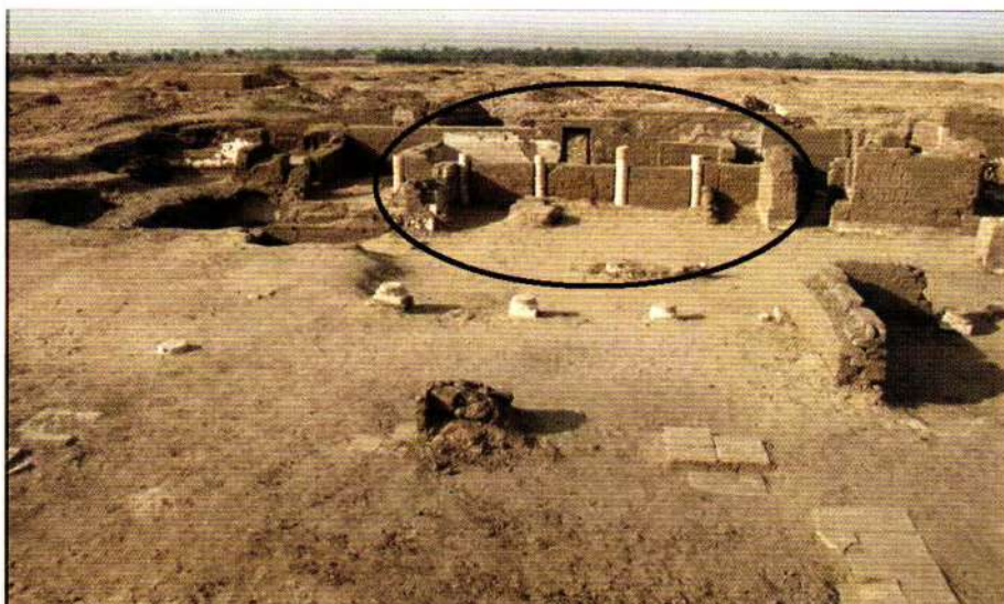
Figs. 1a and b: Extensive damage, looting, and digging was done by the villagers in 2012 to the North Cemetery, called "Mariam" by the villagers. At top is a photo from 2010. The area circled is shown in a detail photo from October 2012 at bottom. The columns have been overturned and many holes have been dug. Damage like this was done to the entire North Cemetery Area.
