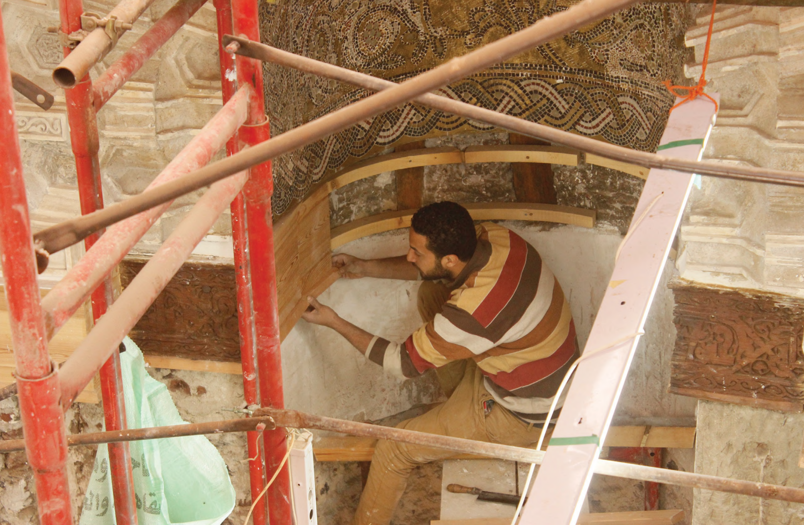
Top: Carpentry work on the lower frieze
