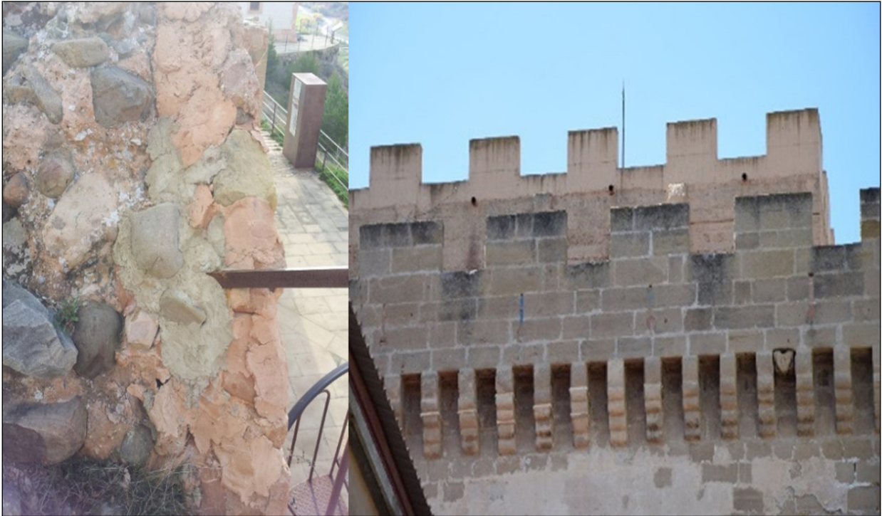
Figure 3. Different uses for concrete: left: Crown in Anguciana; right: Wall in Herce (author).
