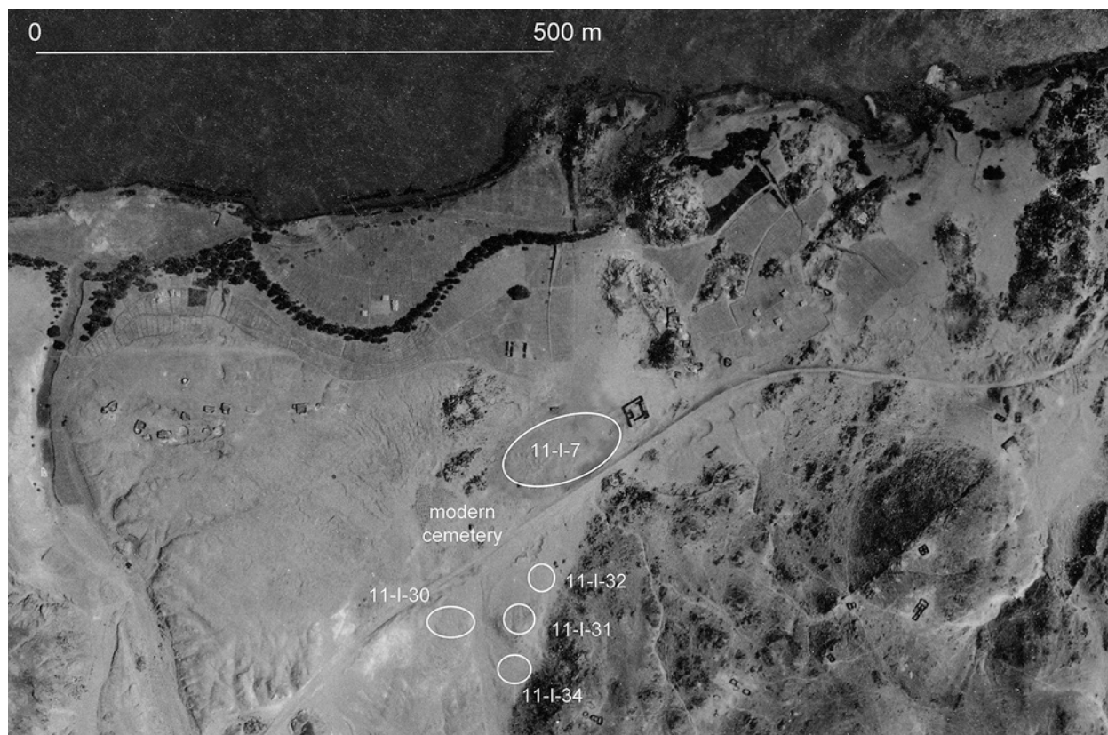
Figure 2.17 Location of [11-I-7 = FNE 39], [11-I-32 = FNE 41] and [11-I-34 = FNE 44] and nearby sites in Sigaga plain, west of Murshid.
