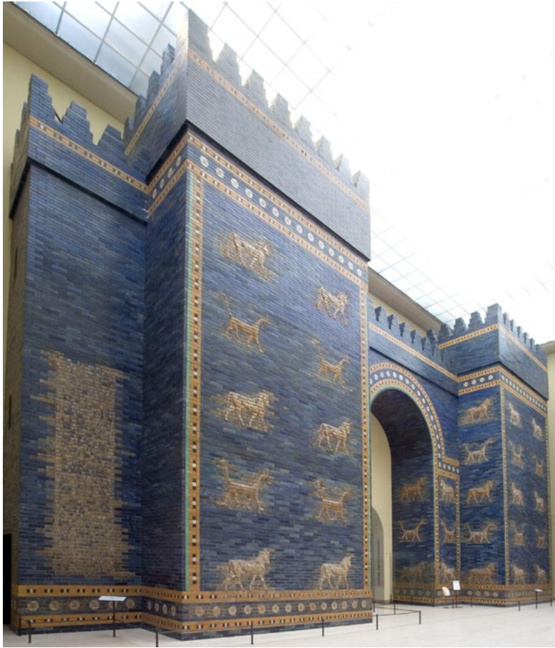
Figure 10. Ishtar Gate, VAM reconstruction with glazed animal reliefs. Ancient fragments with glazed animal reliefs fill about 20% of the surface, i.e. 26 bulls ( rīmu ), 16 dragons ( mušḫuššu ), one inscription, and part of the lowest decorative frieze. Vertical distance between animal feet is 2.0 m. Cf. Figure 11 (© Vorderasiatisches Museum, SMB, photo: Olaf M. Teßmer).
