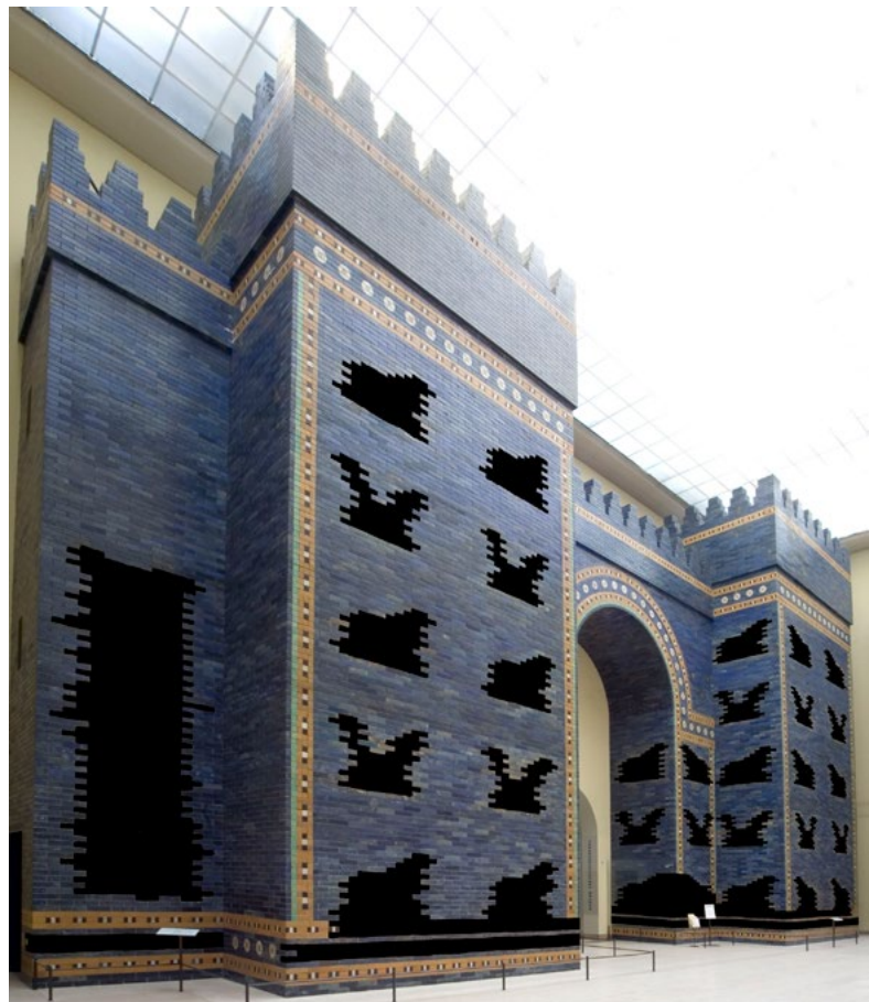
Figure 11. Ishtar Gate, the reconstructed gate at the VAM, cf. Figure 10, with all parts reconstructed with ancient fragments in black. All the remaining parts in full colour, i.e. about 80% of the surface, including all upper parts and all backgrounds are of modern bricks made in the 1920s (© Vorderasiatisches Museum, SMB, photo: Olaf M. Teßmer; black by author).
