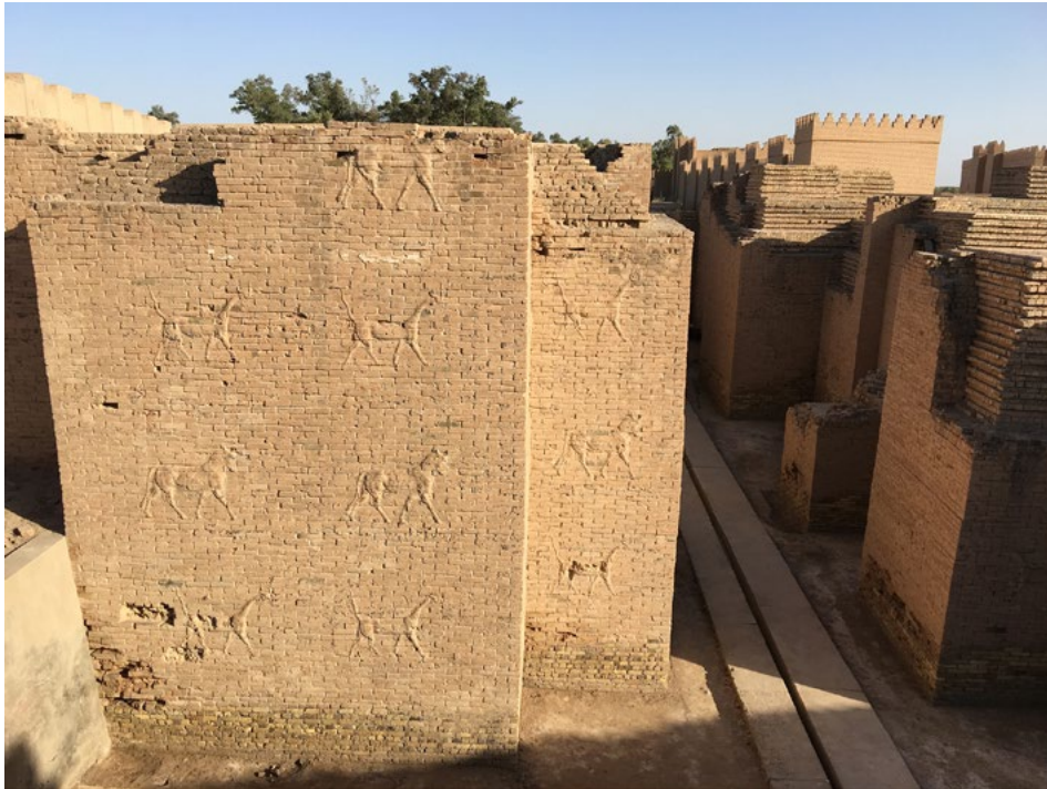
Figure 4. Unglazed baked clay bricks with reliefs. The Ishtar Gate in Babylon in situ . Bulls ( rīmu ) and dragons ( mušḫuššu ). Unusually good light conditions at dusk. In daylight conditions the reliefs are much less visible. The vertical distance between the feet of the animals is 2.0 m. May 2017.
