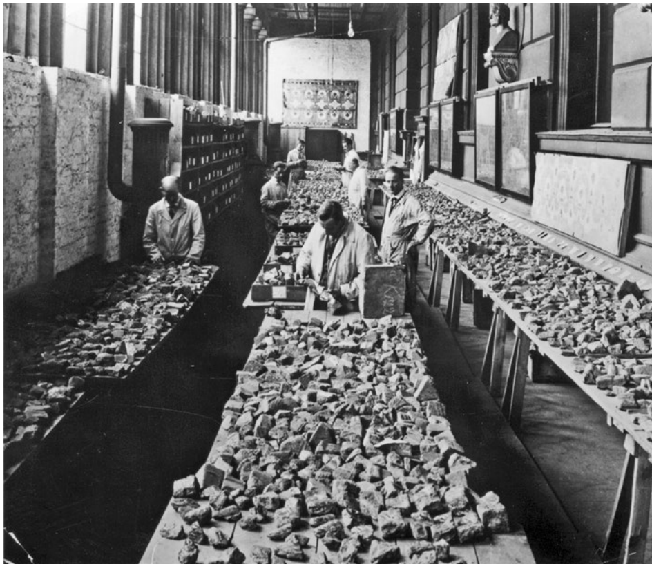
Figure 2. Ishtar Gate fragments in the 1920s, VA. Reconstruction of glazed bricks from fragments. The working room is now the portico in front of the Neues Museum, Berlin. PhBab 3700 (© Vorderasiatisches Museum, SMB).
