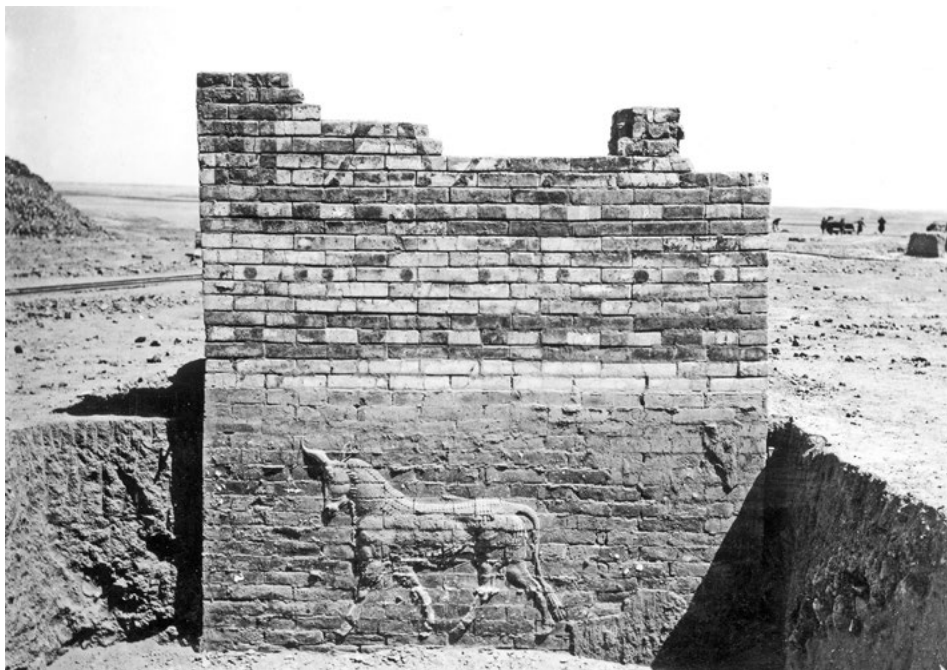
Figure 7. Flat, glazed brick decoration, Bab 20641a, with legs of a bull ( rīmu ) over unglazed bull relief. Before the excavations the terrain was about 2 m above the top of the wall remains. April 1902. PhBab 159 (©Vorderasiatisches Museum, SMB / Deutsche Orient-Gesellschaft).
