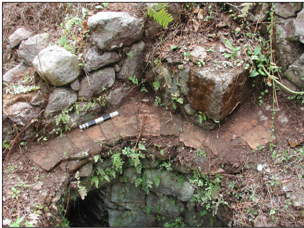
Figure 3.10. Upper Rawlins: boiling house, ceramic tiles in situ (19), surrounding the 'copper' setting, from SE
