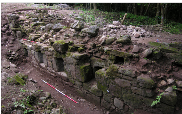
Figure 3.8. Upper Rawlins: boiling train showing stoke-hole apertures and vents above, from SW
