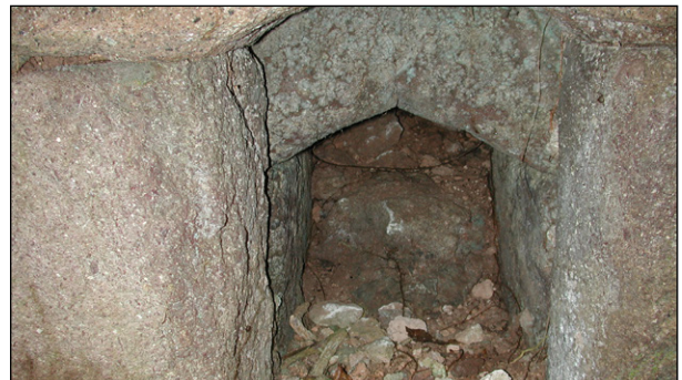
Figure 3.16. Upper Rawlins: blocked flue in boiling train, showing conversion from Spanish to Jamaica train
