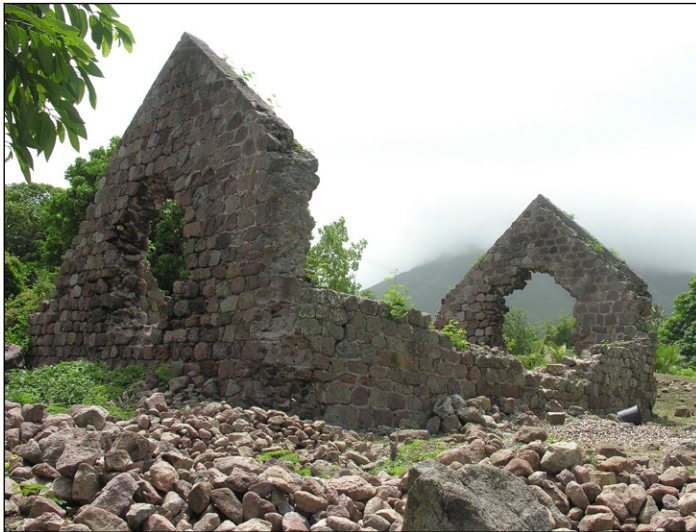
Figure 2.1. Fenton Hill: boiling house (B) from SE
