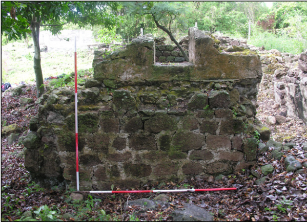
Figure 2.17. Fenton Hill: Structure A, E wall from outside showing window in gable and offset wall for gutter
