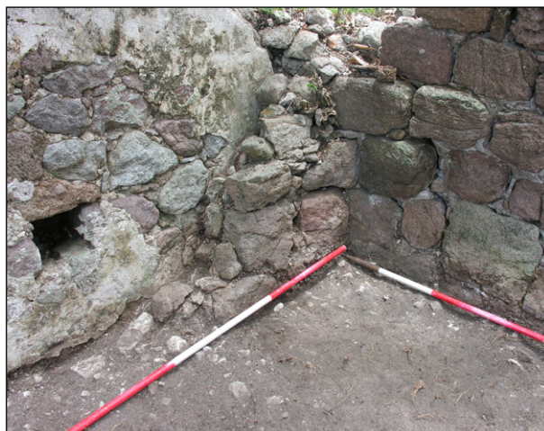
Figure 2.21. Fenton Hill: SW corner of Structure A, showing overlapping wall, and drain hole in wall, from NE
