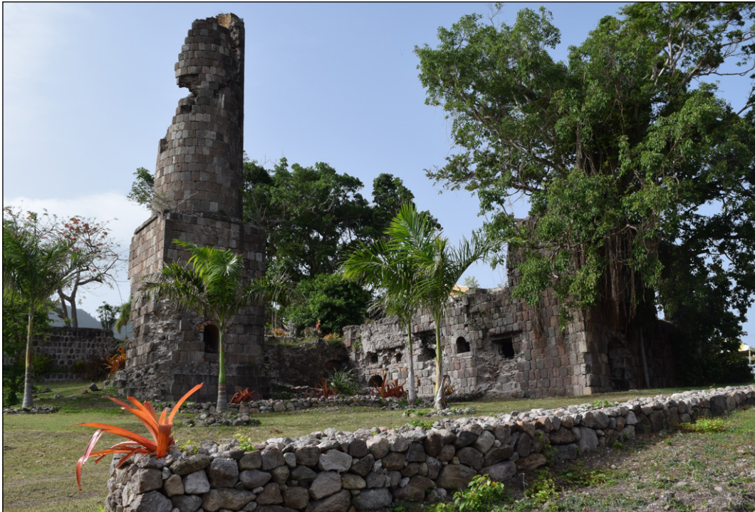
Figure 4.3. Fothergill's: remains of the chimney and boiling house (photograph: Robert Philpott, 2018)
