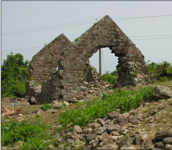
Figure 2.9. Fenton Hill: boiling house (B) from N
